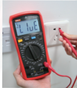
Live and nature wires identification
